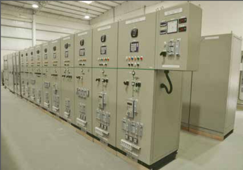
33kV Combined Control & Relay Panels at Aziaba North-3 Primary Station for MEDC, Oman
