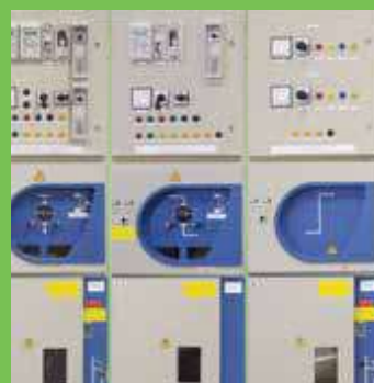
MV Power distribution
