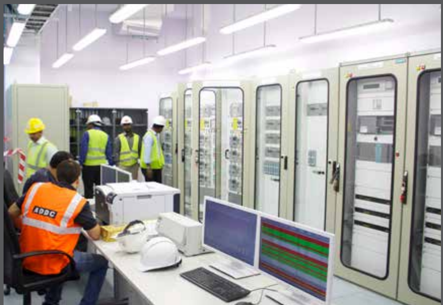
12MVAR, 22kV Capacitor Bank Control & Protection Panel SAT testing for ADWEA, UAE
