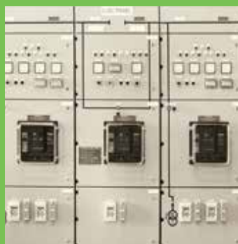
LV Power distribution
